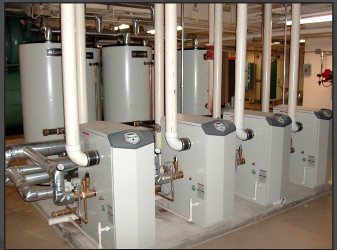
INSTALLED ARMOR & LOCK-TEMP TANKS
