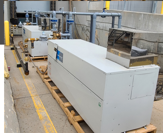
» ABOVE: INSTALLED COPPER-FIN2
