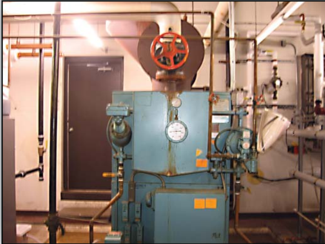
Two 98% thermal efficient Sync boilers carry the load of the building and an existing boiler remains as a back-up boiler.
