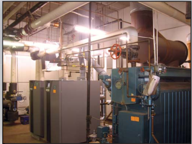
Two 98% thermal efficient Sync boilers carry the load of the building and an existing boiler remains as a back-up boiler.
