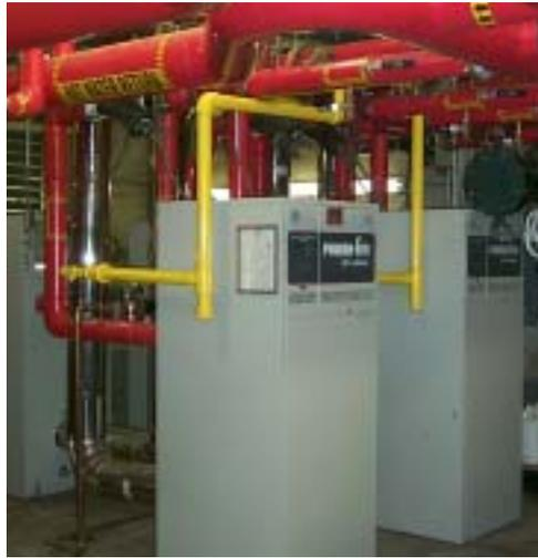
Atlantis Services chose to install four Lochinvar Power-Fin® (PBN1700) boilers, which were compact enough to fit in the floor space of the small mechanical room and deliver the Btu's needed to fulfill the heat load. The four boilers deliver a total of 5,916,000 Btu/Hr output in the same space previously occupied by two boilers with approximately 2,500,000 Btu/Hr output.
