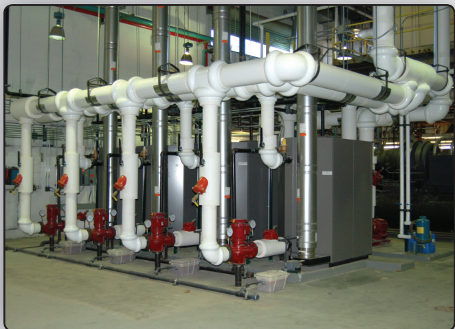
4 CREST Boilers in place of the Old Steam Boilers
