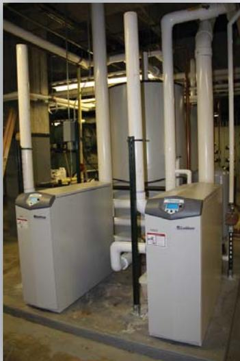
traditional water heater to fail in as little as two to five years and substantially increase operating costs. For example, just 1/4-inch of scale in the tank can increase operating costs by as much as 25 percent. Since ARMOR heats the water and then deposits it in an unfired storage tank, lime scale buildup does not impair the heat transfer efficiency.
