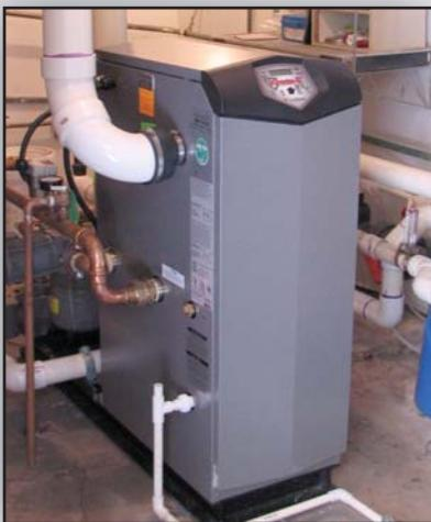
Local installer, Ballard's Plumbing and Heating was contracted to install the Aquas and the installation proved easier than anticipated. First, the Aquas Package took less floor space than the original pool heater. The original metal vent pipe was replaced with easy to install 4" PVC. PVC pipe was also used for the combustion air which supplied the boiler with clean air, free of destructive pool chemicals. The simple water piping routed pool water straight through the Aquas pool heat exchanger.
